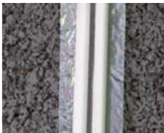
Fig. 36 Metallic tape can be used to aid electronic pipe detection
