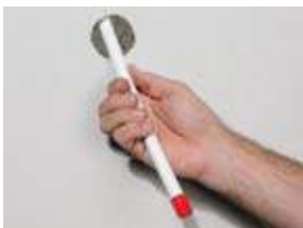
Fig. 22 Always protect pipe ends
