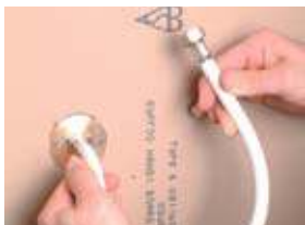
Fig. 48 Installation of HX102 terminal fitting plate and HX101/15, 15mm conduit terminal
