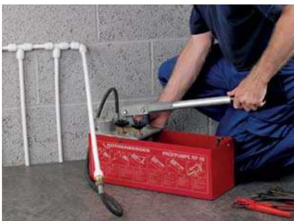
Fig. 57 Pressure testing
