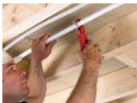
Measure and cut in-situ
