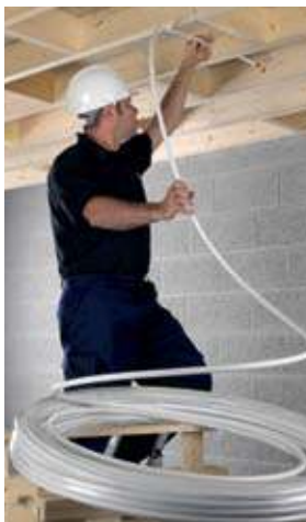
Fig. 21 Packaging retains pipe until last metre
